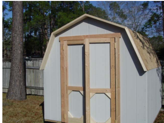
Front Fly Rafters Installed
