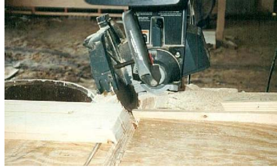
Sawing the fly rafters
