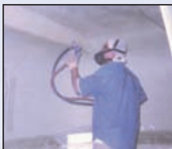
Marine adhesives being applied for wall coverings.
