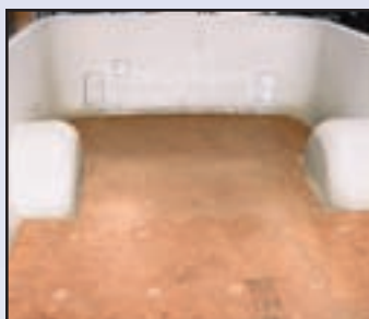
Wood flooring installed and sealed with fiberglass prior to carpeting.
